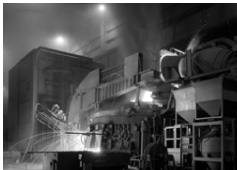
Electric Arc Furnace (EAF) transformation
