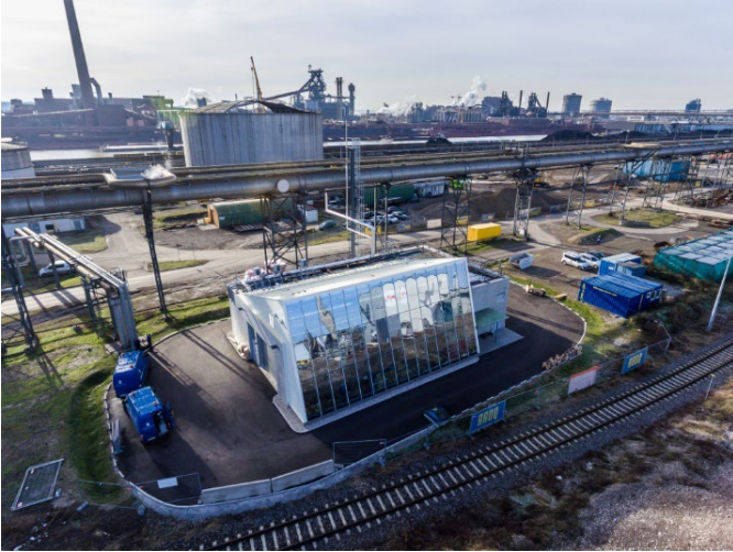
H2Future demonstration plant Industrial scale PEM electrolyser for hydrogen production with dynamic response for all kinds of grid services
