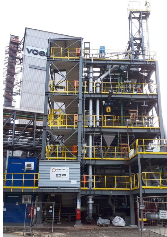
HYFOR pilot plant Direct reduction of ultrafine iron ores with hydrogen in a fluidized bed process
