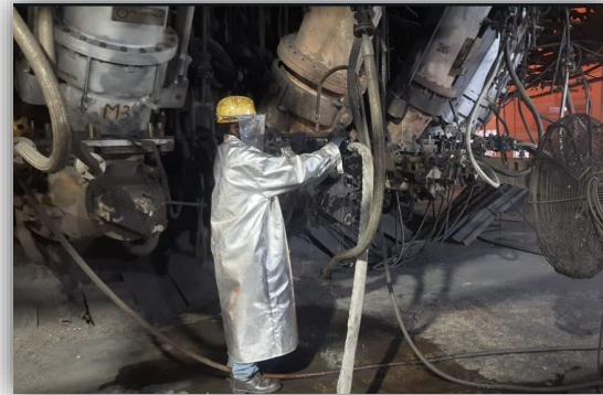
Injection setup in blast furnace
