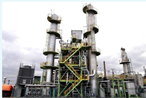
Commercialized plant No.1 (AIR WATER CARBONIC INC.)
