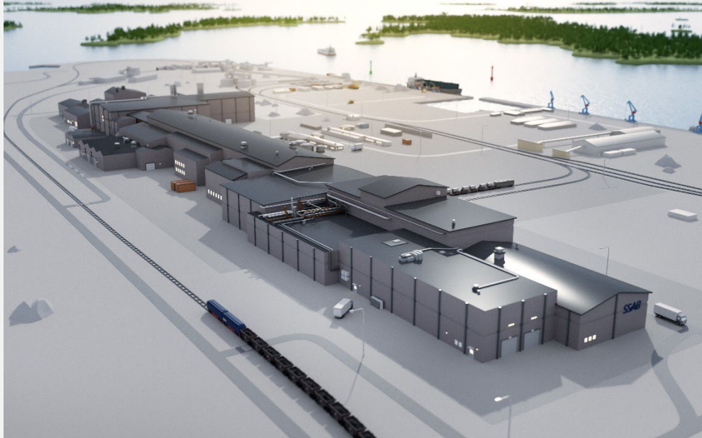
Planned new steel mill in Luleå, Sweden
