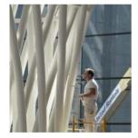
To prevent steel framing's load-bearing capacity from diminishing at excessive temperatures, steel structures are coated with a
