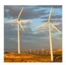
A wind turbine is comprised of between 84% and 90% iron and steel materials, used in the tower, nacelle and rotor. An average of
