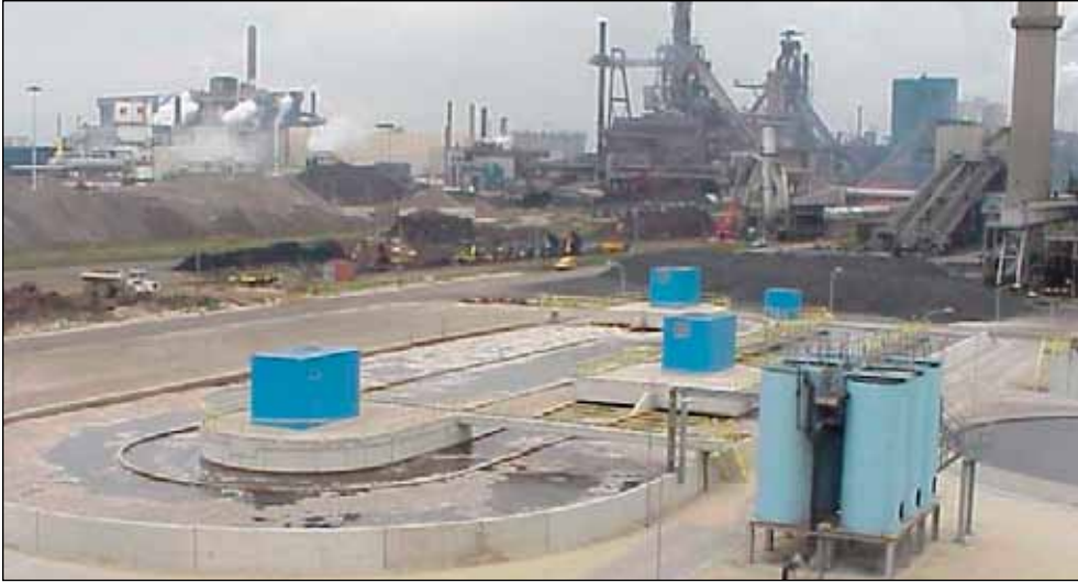
Figure 1.3.1 The new biological treatment plant
