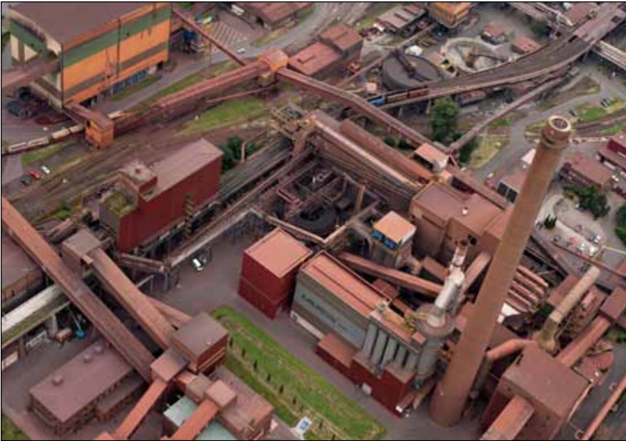
Figure 4.1.1 voestalpine Stahl, Sinter plant
