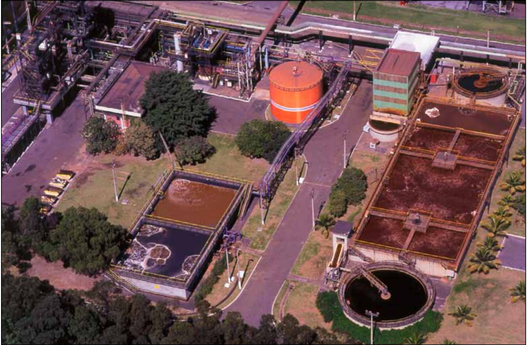
Figure 1.2.2 Overview of ArcelorMittal Tubarão coke plant wastewater treatment
