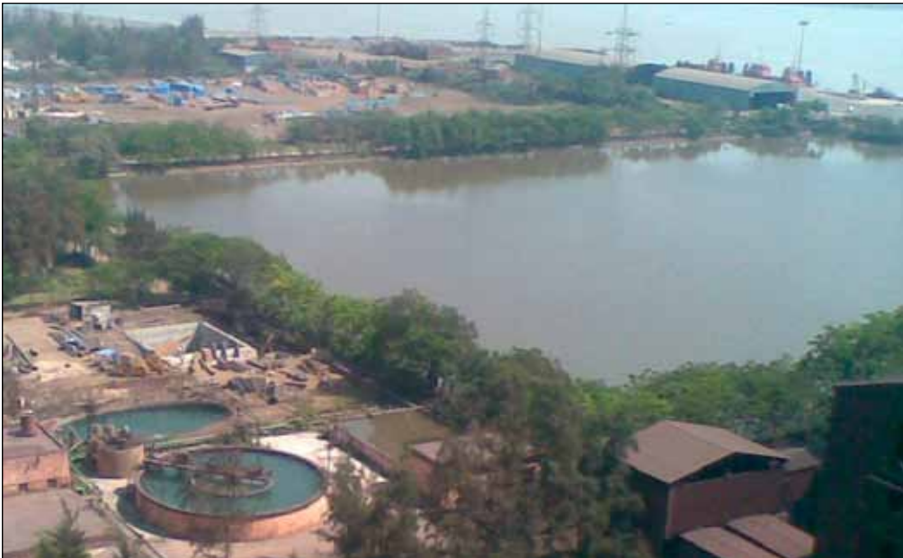
Figure 9.2.1 Raw water treatment plant and reservoir
